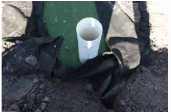
Figure 16 (Below): Cut an "X" into Biaxial Mesh to accommodate pipe penetration
