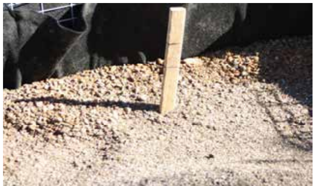
Figure 22: Place biofiltration soils, being careful not to mix with any other site soils, to specified depth
