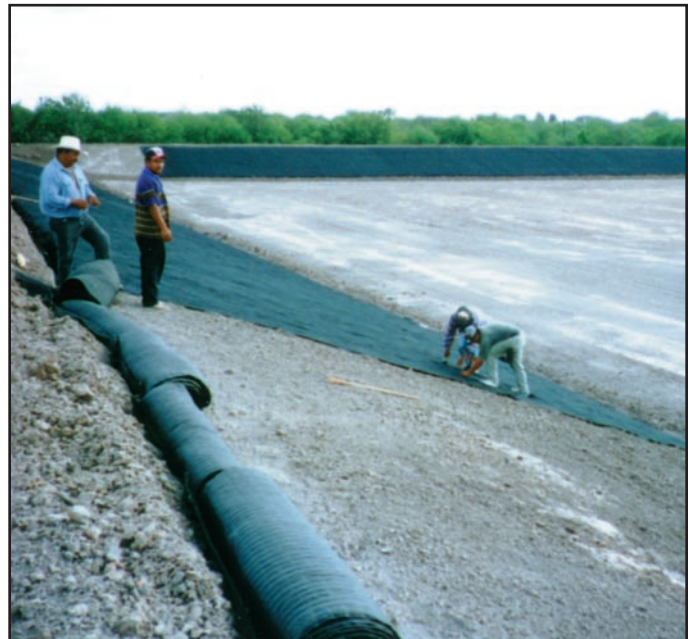
Installation of Landlok ® TRM 1061B
