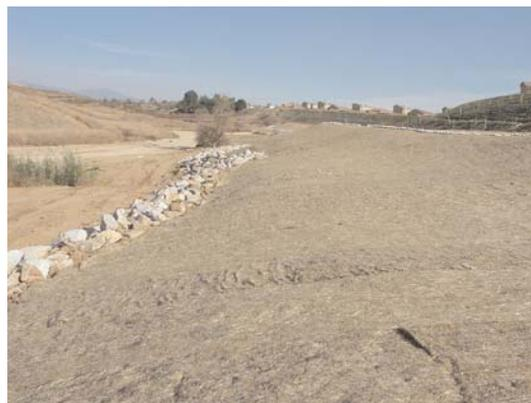
Landlok® TRM 450 Turf Reinforcement Mat was placed in a side tributary channel to Marshall Creek. This tributary conveyed water from a storm drain pipe from the Three Rings Ranch development. This tributary was designed as a bioswale Post Construction BMP; the Landlok TRM 450 was used to protect the bioswale from erosion in large storm events.
