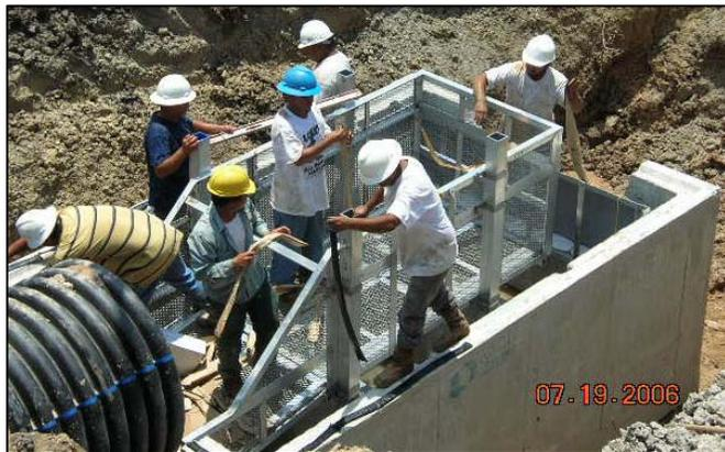
Above: An NSBB being installed. From this image you can see the large metal screen where debris, vegetation, and floatables are collected.
